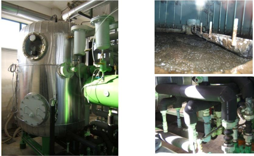
**Figure 3.4** On the left the anaerobic digester and, on the right, the scrapers internal detail and the piping extraction system.
