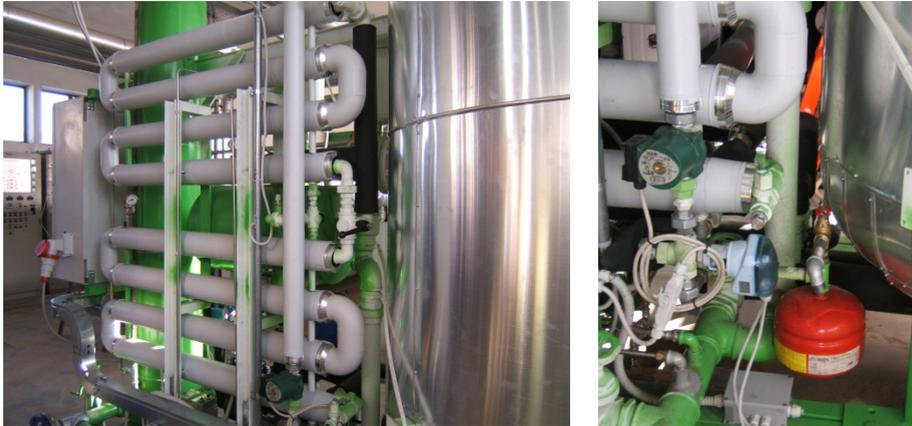
**Figure 3.3** The double-pipe heat exchanger on the left and, on the right, the temperature regulation system and the expansion vessel.
