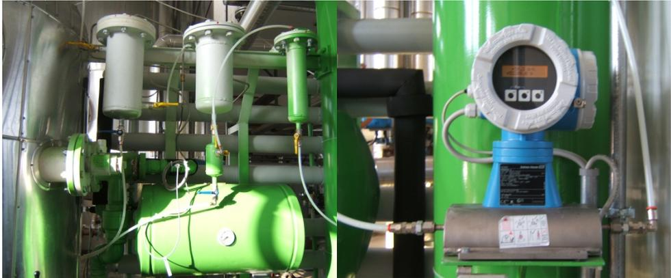
**Figure 3.5** The biogas line columns and, on the right, the flow meter.
